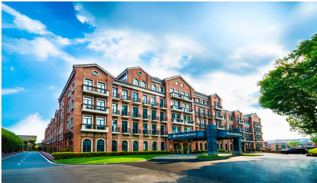
Taoxichuan Traders Hotel whole building view
